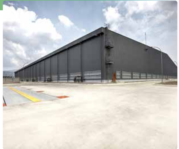
Warehouse in Krakatau Industrial Estate Cilegon
